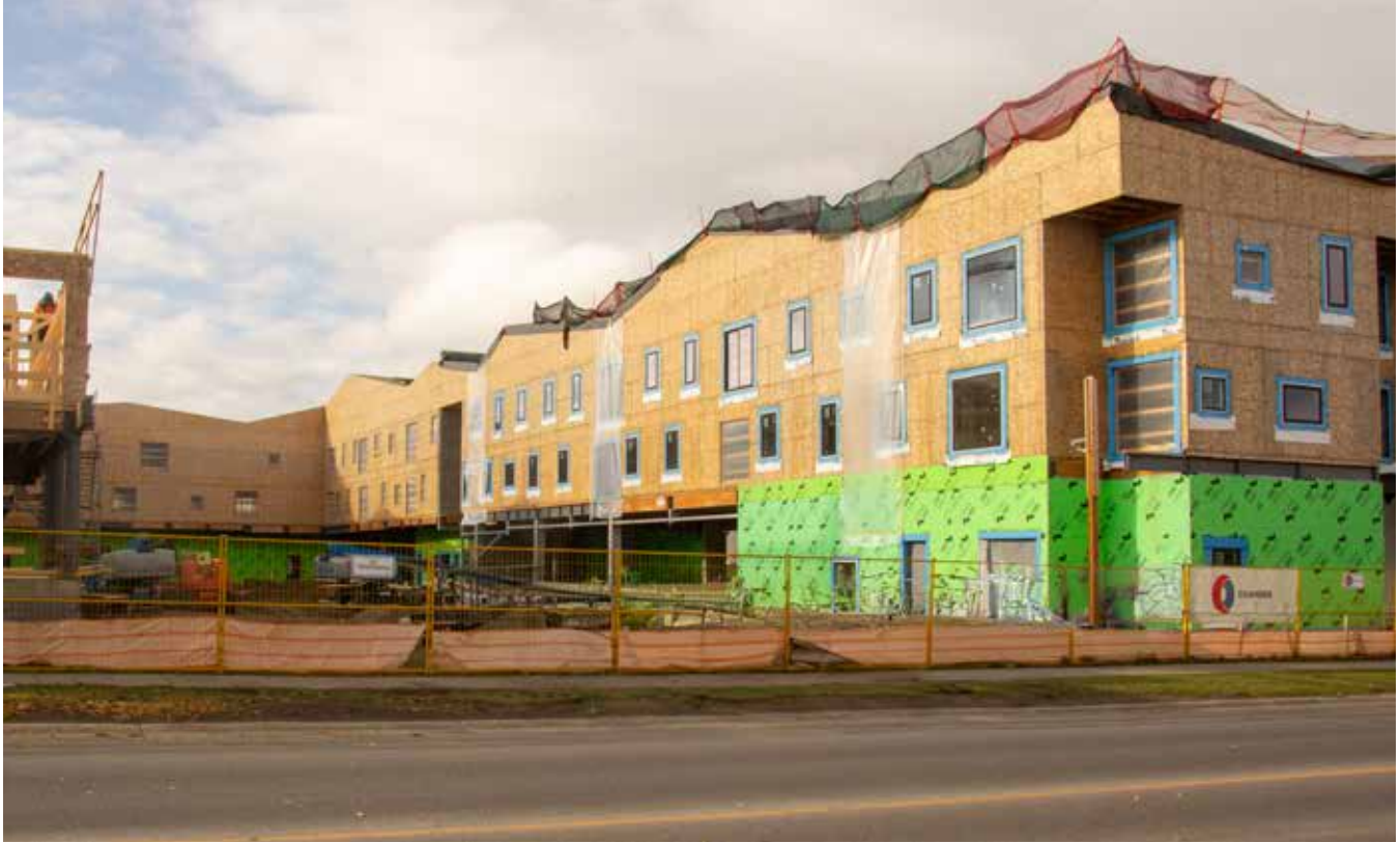
Rundle Manor redevelopment under construction, September 2023.
